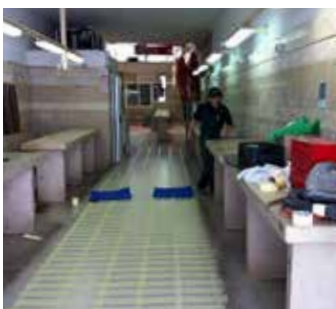
Tiled floor before
