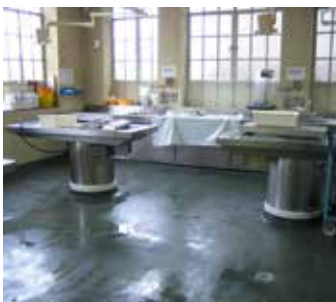
Concrete floor before
